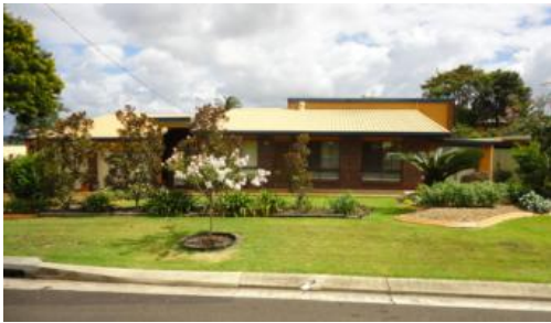
23 Cunningham Crescent, Nambour
