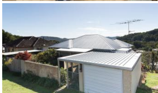
45 Lamington Terrace, Nambour
