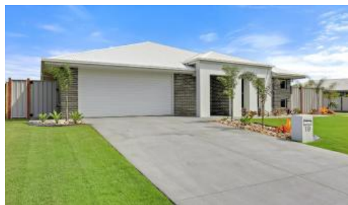
19 Seahaven Cct, Pialba
