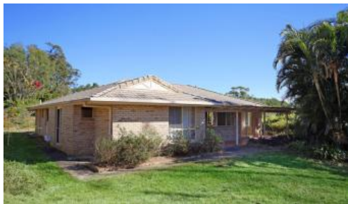
13 Curlew Crescent, Cooroy
