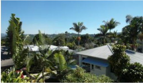
8, 5 Vernon Street, Nambour
