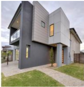
7 Reserve Court, Murrumba Downs
