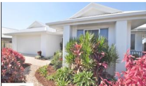
18 Rawlins Crescent, North Lakes
