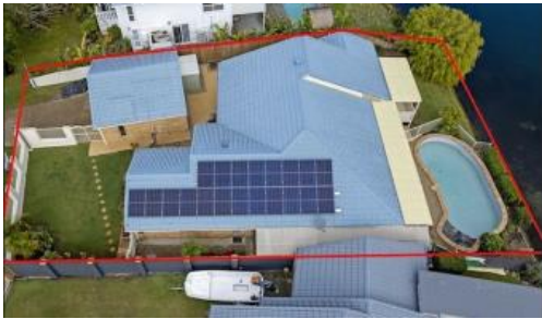
76 Lamerough Pde, Pelican Waters
